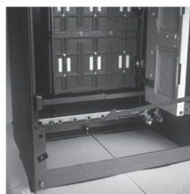
FIGURE 8.7 Horizontal ground bus bars in an MCC.
