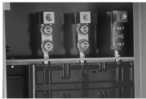
FIGURE 8.8 Source or utility connection, incoming power lugs.
